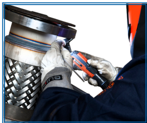
HOSE & FAB WELDING
